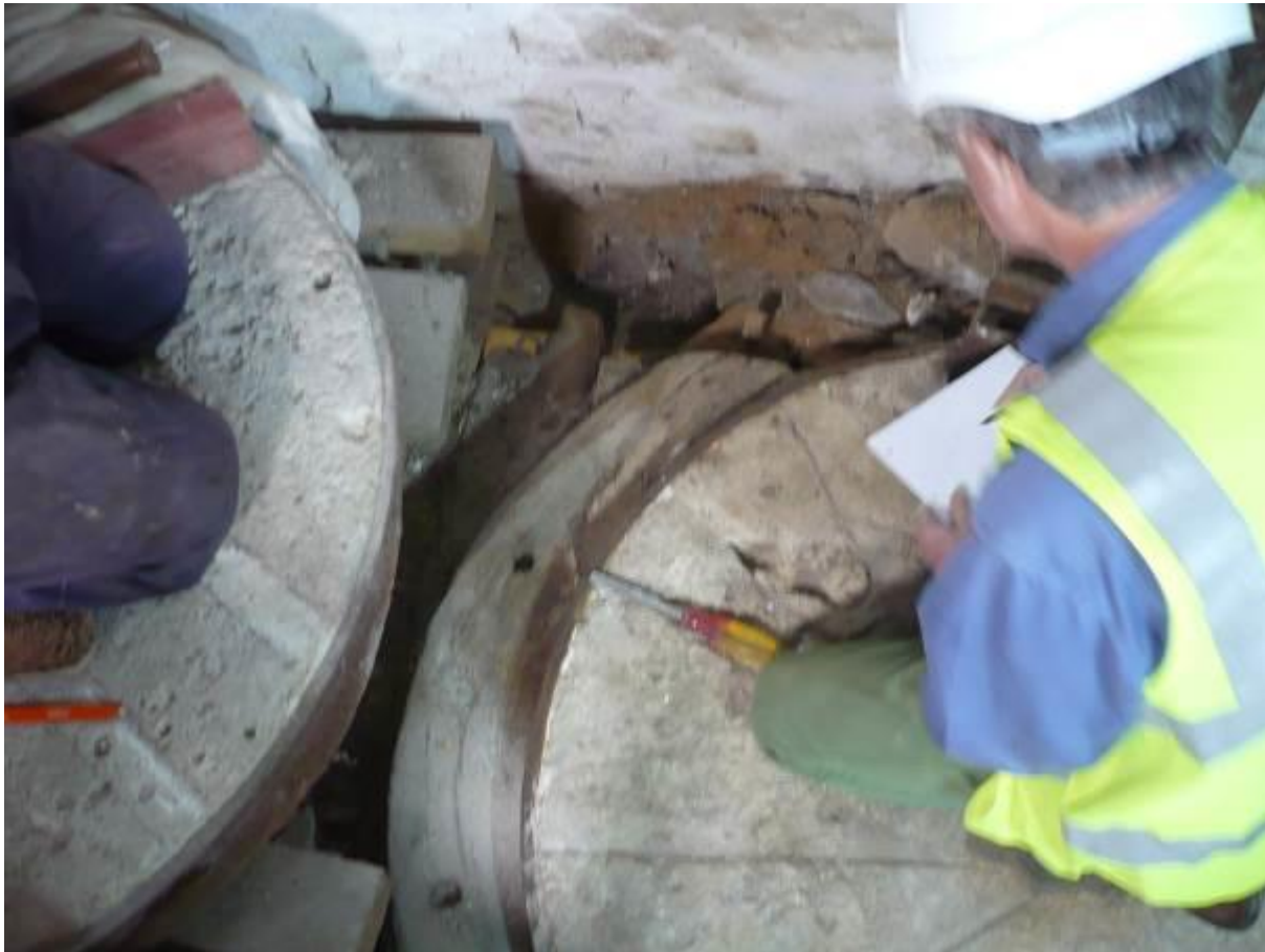
15b Inspection of the rotten timbers of the hurst frame by the outer wall.
