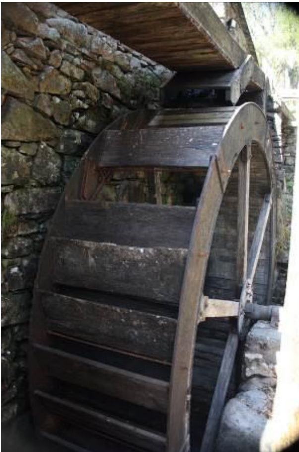
12 Upper wheel showing a crack in the cast rim section. 12a The waterwheel with rotten paddles April 2016.
