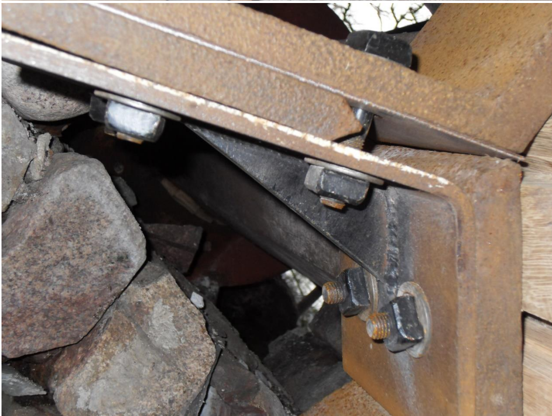
16a and b A repair section after being strengthened by the millwrights.
