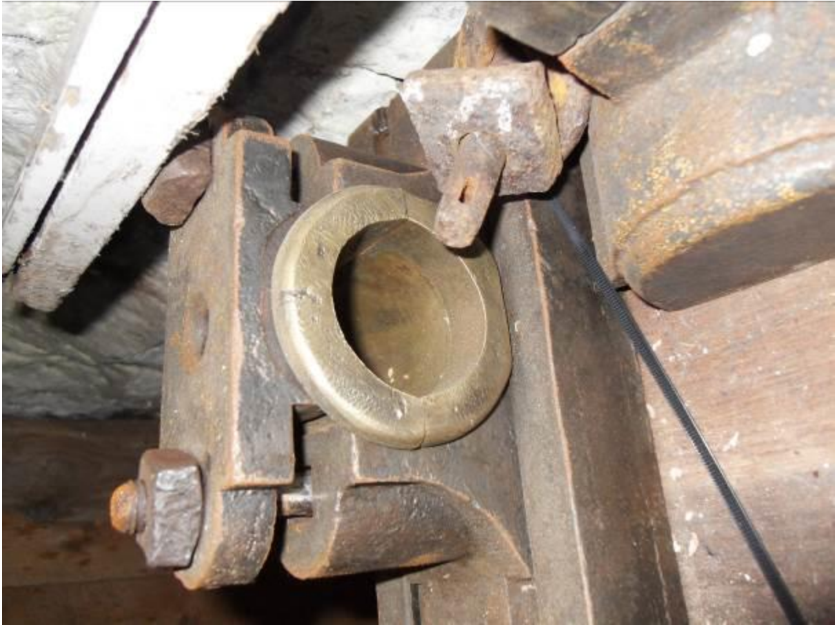
8 An example of a new bronze/brass bearing shell in its block.
