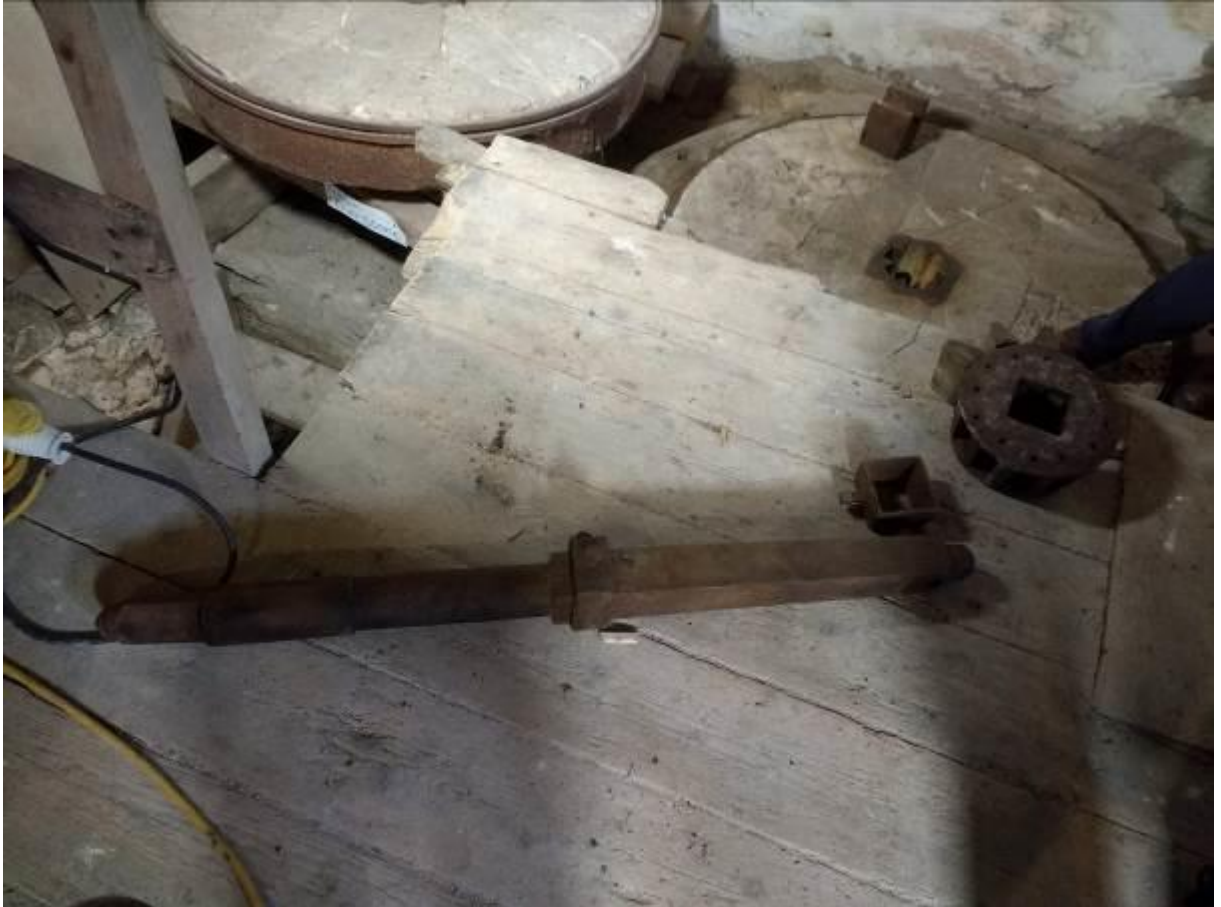
13 The lower millstone shaft and stone nut prior to alteration
