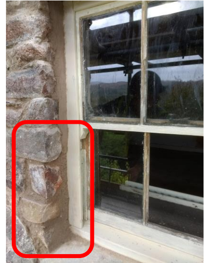
Left hand side image: western jamb to window no. 5 showing area of brickwork covered in cement, 14 th July 2016.
