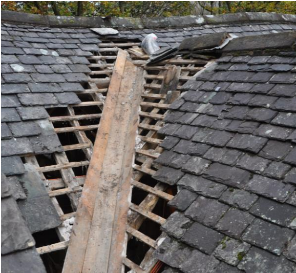
Left hand side image: northern valley gutter under construction, image kindly supplied by Maurice Steele. Right hand side image: finished southern valley gutter. 6 th November 2018
