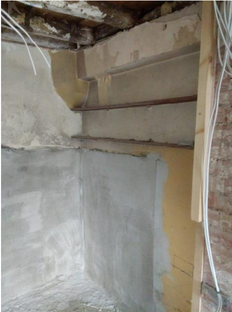
Left hand side image: tanking to north wall and return to living room. Right hand side image: dry lining to kitchen area showing the tanking below and the first fix of electricity. 22 nd November 2018
