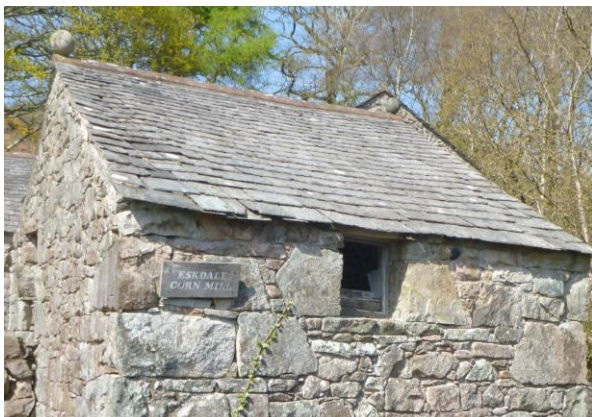
South pitch to stable/hayloft. Left hand side image taken on 5 th May 2016. Right hand side image taken on 26 th October 2018, showing the new roof overhanging the western gable
