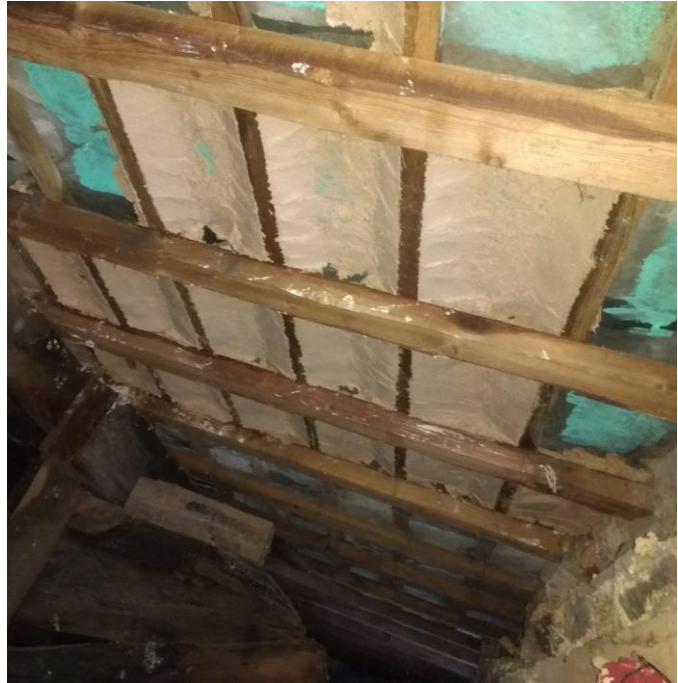
Images of the torching to the underside of the roof above the Drying Room, 22nd November 2018
