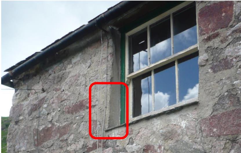
Left hand side image: western jamb to window no. 5 showing area of brickwork covered in cement, 14 th July 2016.
