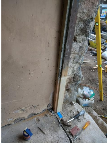
Left hand side image: splice of splice joint between new bottom timber section and existing door frame to front door, 22 nd November 2018. Right hand side image: image showing the refurbished door frames on 13 th December 2018
