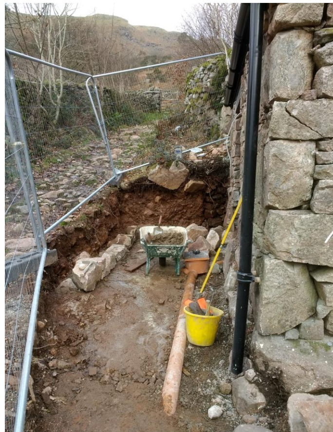
Image of the setting out of the retaining wall, 13 th December 2018
