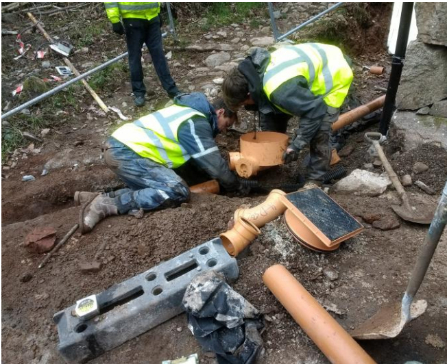
New foul drainage system to the wheelchair accessible toilet, 22 nd November 2018
