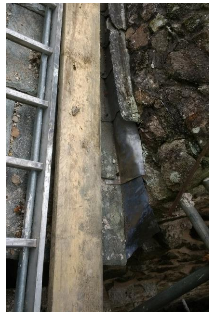
Abutment between the Milling Room roof and the southern gable of the Drying Room. Left hand side image taken on 6 th September 2018. Right hand side image taken on 6 th November 2018
