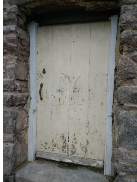
Left hand side image: splice of splice joint between new bottom timber section and existing door frame to front door, 22 nd November 2018. Right hand side image: image showing the refurbished door frames on 13 th December 2018
