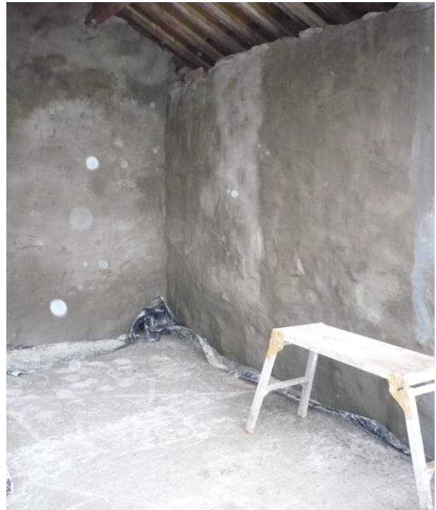
Image of the concrete slab to the cart shed and the tanking to masonry wall on 26 th October 2018
