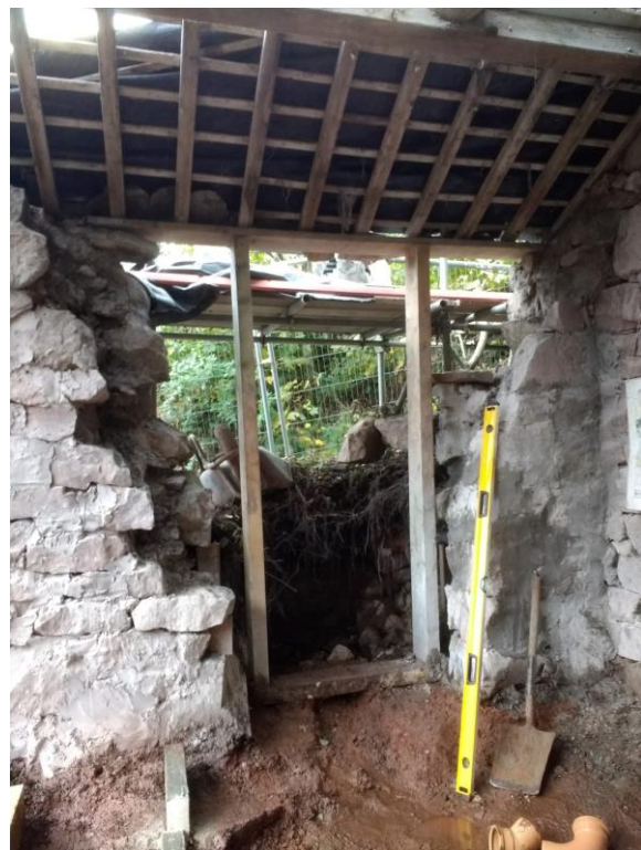
Left hand side image: general image of the cart shed with the western pitch stripped off, the ground floor excavation and the concrete foundation to the new south elevation. Right hand side image: masonry opening for doorway into new wheelchair accessible toilet, 9 th October 2018
