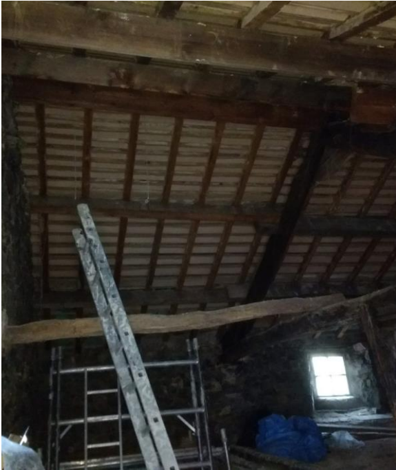
Images of the torching to the underside of the roof above the Drying Room, 22nd November 2018
