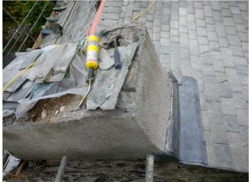
Left hand side image: western chimney with cement flaunching, 6 th September 2018. Right hand side image: western chimney after hacking off the cement flaunching, 9 th October 2018
