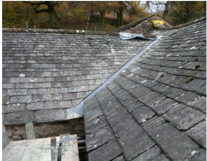
Left hand side image: northern valley gutter under construction, image kindly supplied by Maurice Steele. Right hand side image: finished southern valley gutter. 6 th November 2018
