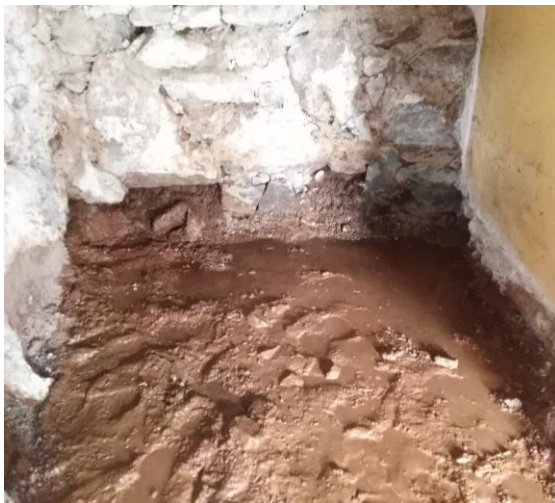
Left hand side image: water ingress at the base of the north wall to the living room, 20 th September 2018. Right hand side image: temporary haunch to the base of the wall preventing water ingress and trench for new internal drain, 9 th October 2018
