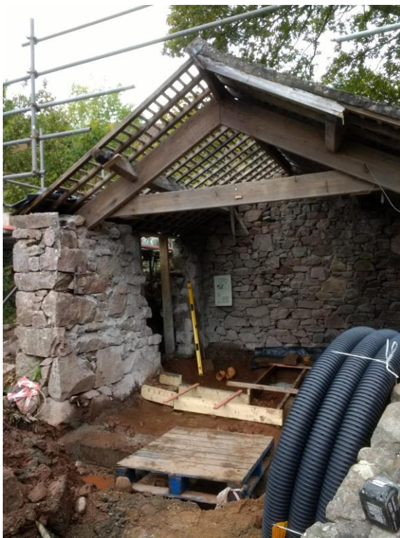
Left hand side image: general image of the cart shed with the western pitch stripped off, the ground floor excavation and the concrete foundation to the new south elevation. Right hand side image: masonry opening for doorway into new wheelchair accessible toilet, 9 th October 2018
