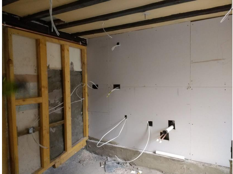
Left hand side image: tanking to north wall and return to living room. Right hand side image: dry lining to kitchen area showing the tanking below and the first fix of electricity. 22 nd November 2018
