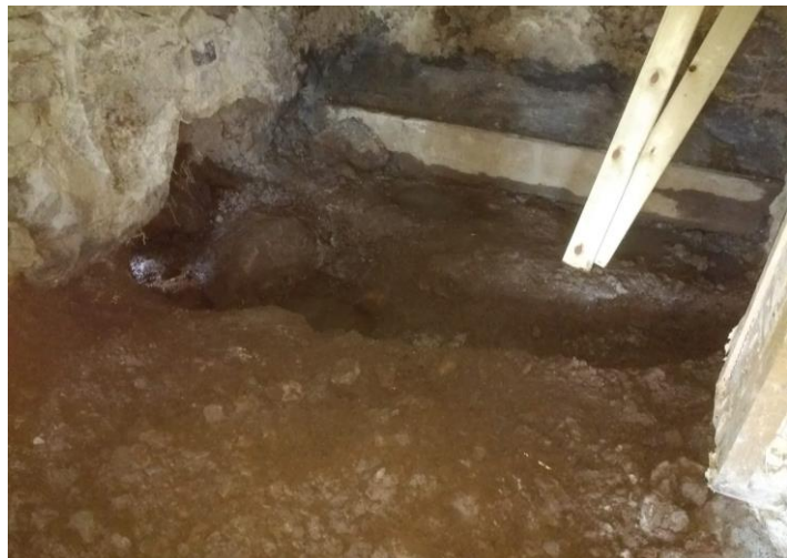
Left hand side image: water ingress at the base of the north wall to the living room, 20 th September 2018. Right hand side image: temporary haunch to the base of the wall preventing water ingress and trench for new internal drain, 9 th October 2018
