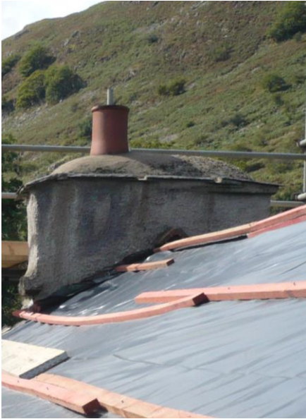
Left hand side image: western chimney with cement flaunching, 6 th September 2018. Right hand side image: western chimney after hacking off the cement flaunching, 9 th October 2018
