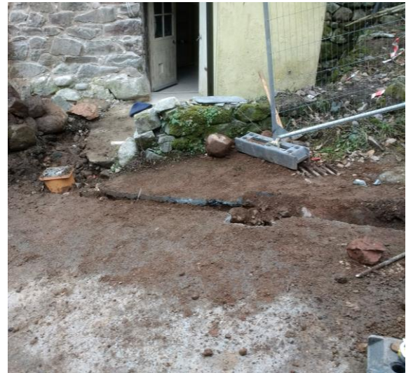
New foul drainage system to the wheelchair accessible toilet, 22 nd November 2018
