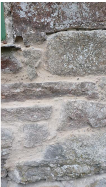
Left hand side image: first sample of lime pointing deemed as unsatisfactory, 7 th August 2018. Right hand side image: sample of approved lime pointing at the top of the eastern gable, 6 th September 2018
