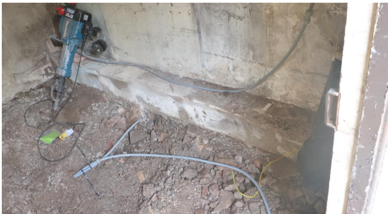
Image showing the concrete haunch at the bottom of the north wall to the kitchen, 7 th August 2018
