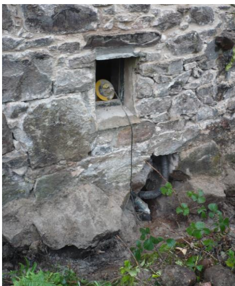
Left hand side image: connection point of the internal drainage to the external French drain (west elevation). Right hand side image: French drain to north elevation under construction, 26 th October 2018
