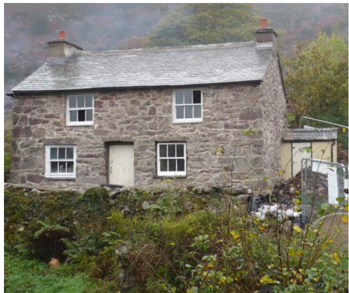
Left hand side image: roof under construction, image kindly supplied by Maurice Steele. Right hand side image: south elevation of the cottage after reroofing and repointing works, 26 th October 2018
