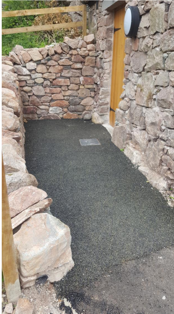
Image of FlexiPave to entrance to wheelchair accessible toilet taken on 4 th July 2019
