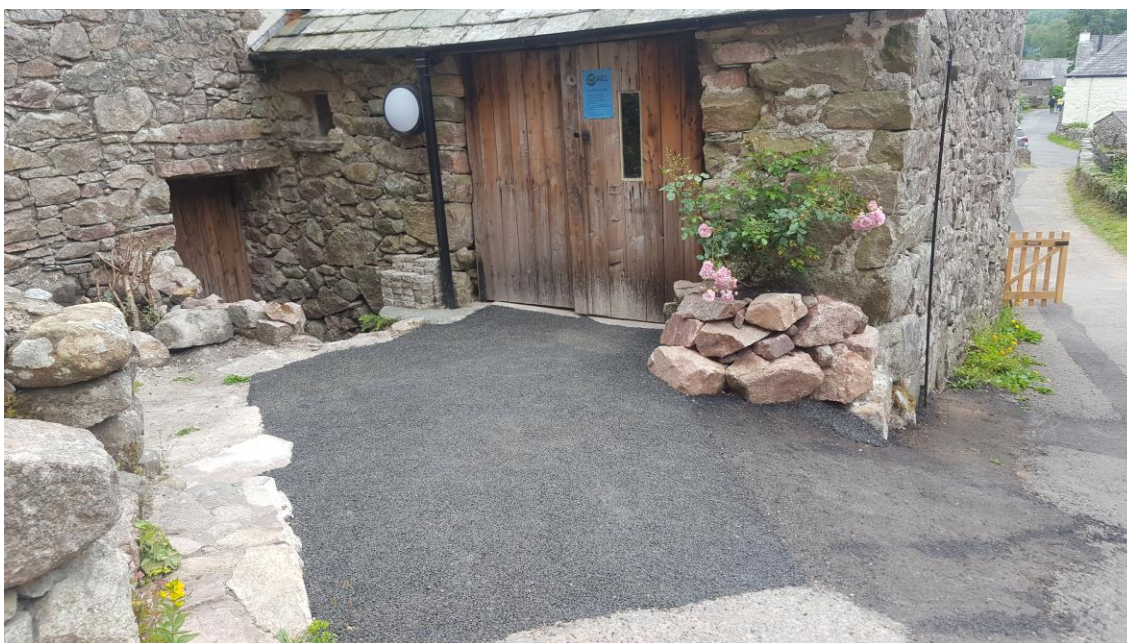
Image of FlexiPave to facilitate access for wheelchair users into exhibition room, taken on 4 th July 2019
