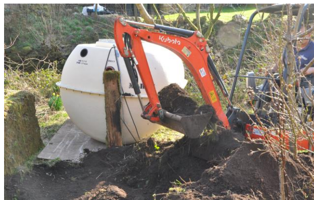
Image of the new sewage treatment plant being installed on 25 th February 2019
